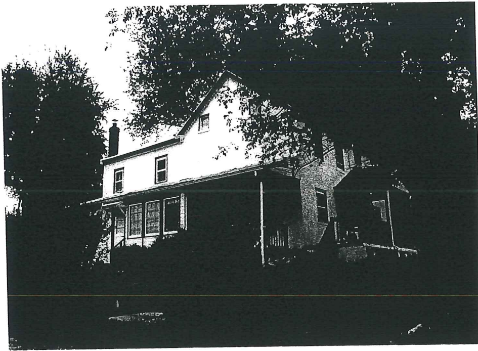
Photograph 2 – Side and main façades of the residence. Note the modern wood balustrades and replacement front porch.
