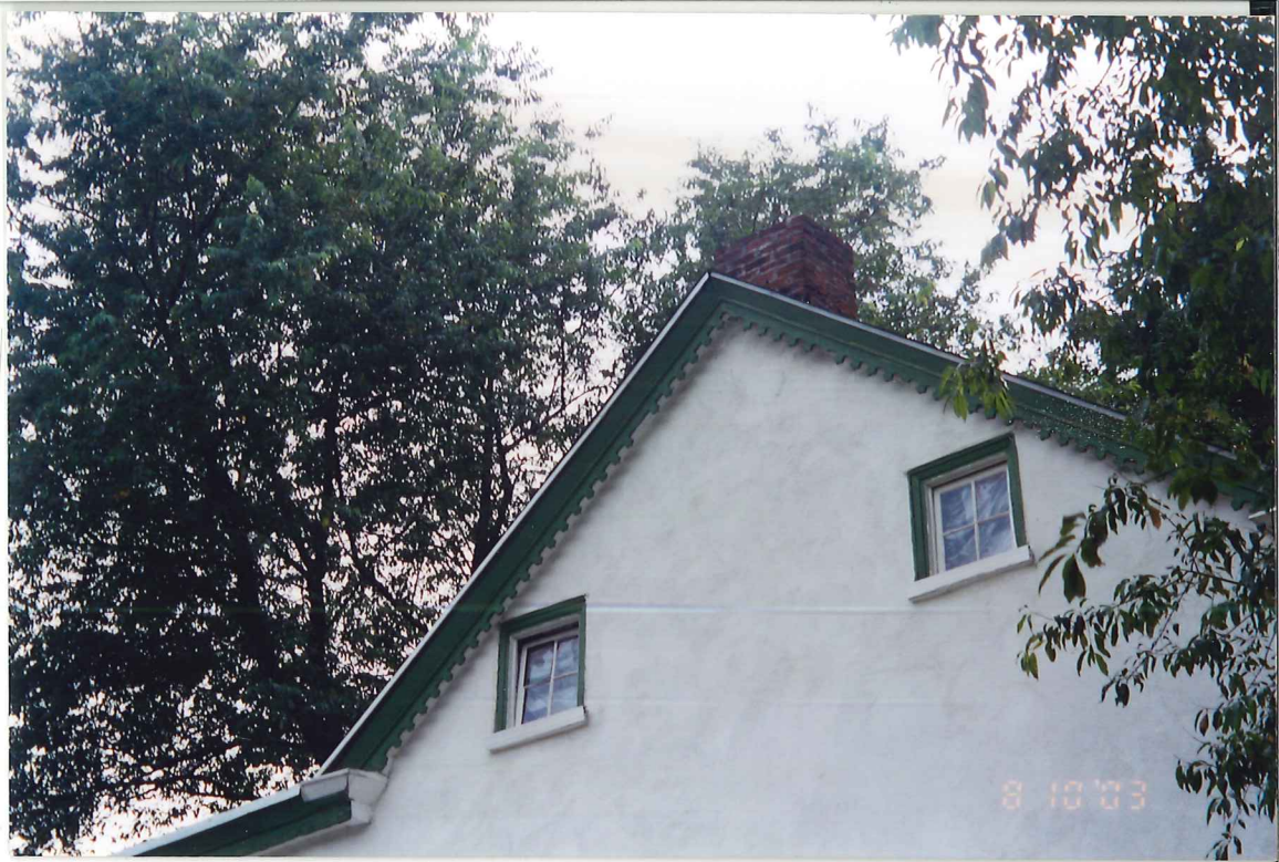
View of eave on east side of house and fireplace in front room.
