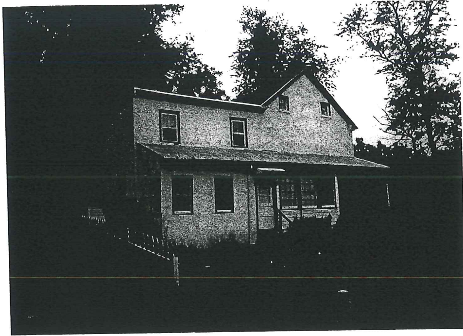
Photograph 4 – View of the rear and side facades of the residence. Note the rear extension and side porch additions.
