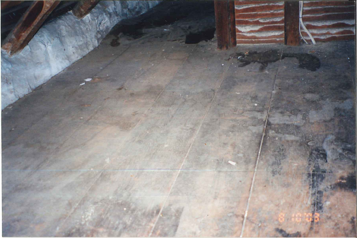
Old wide floor boards in attic & door to second room.
