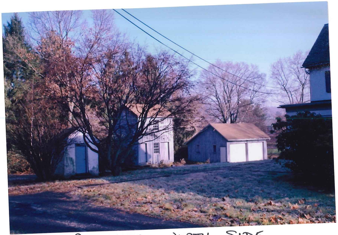
OUT BUILDINGS NORTH SIDE
