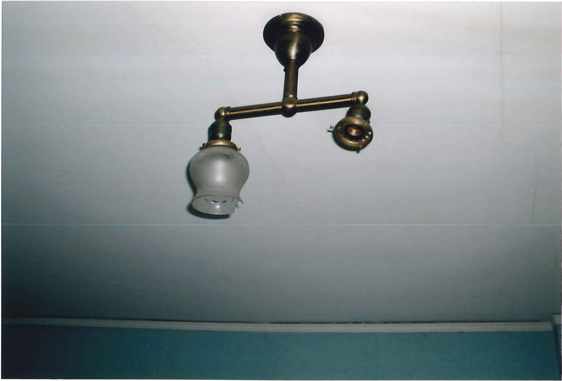
OLD STYLE - LIGHT FIXTURE REAR (NORTH) BEDROOM
