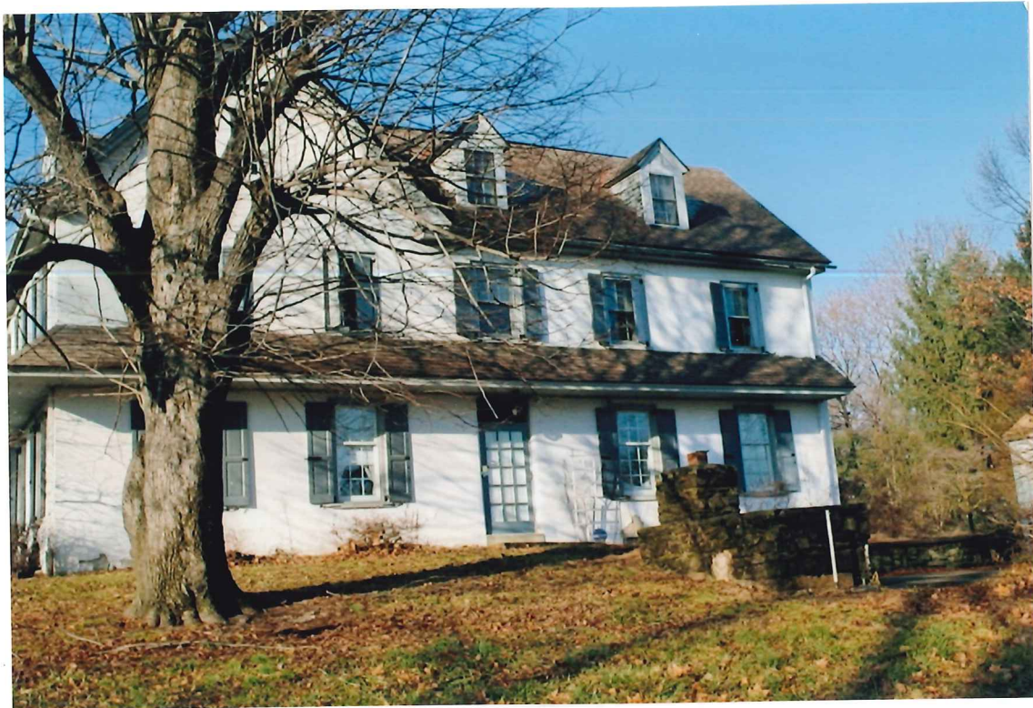
EAST SIDE - TOWARDS ROAD
