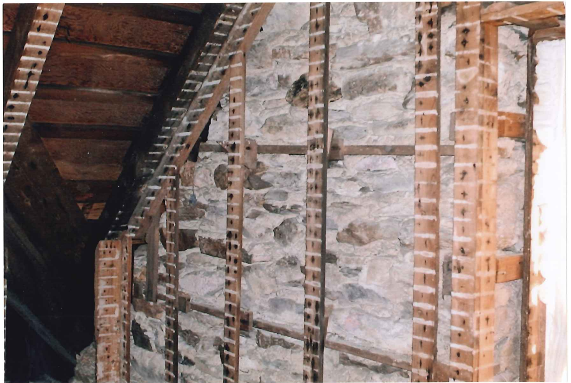
ATTIC - WALLS OF STONE
