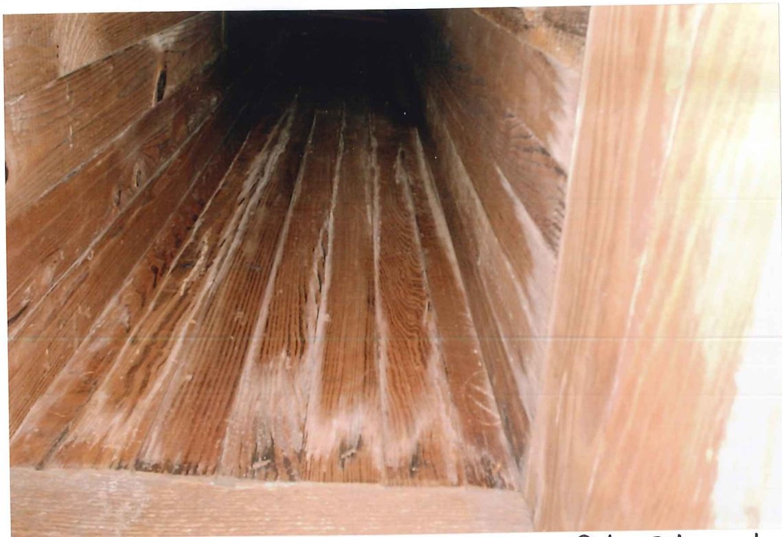
LOOKING UP THE LAUNDRY SHUTE! THIS WAS A HOUSE OF LUXURY .
