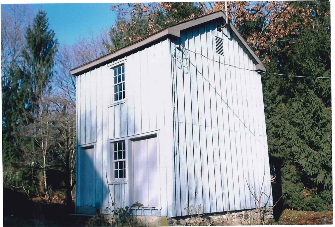
RUBBLE STONE FOUNDATION
