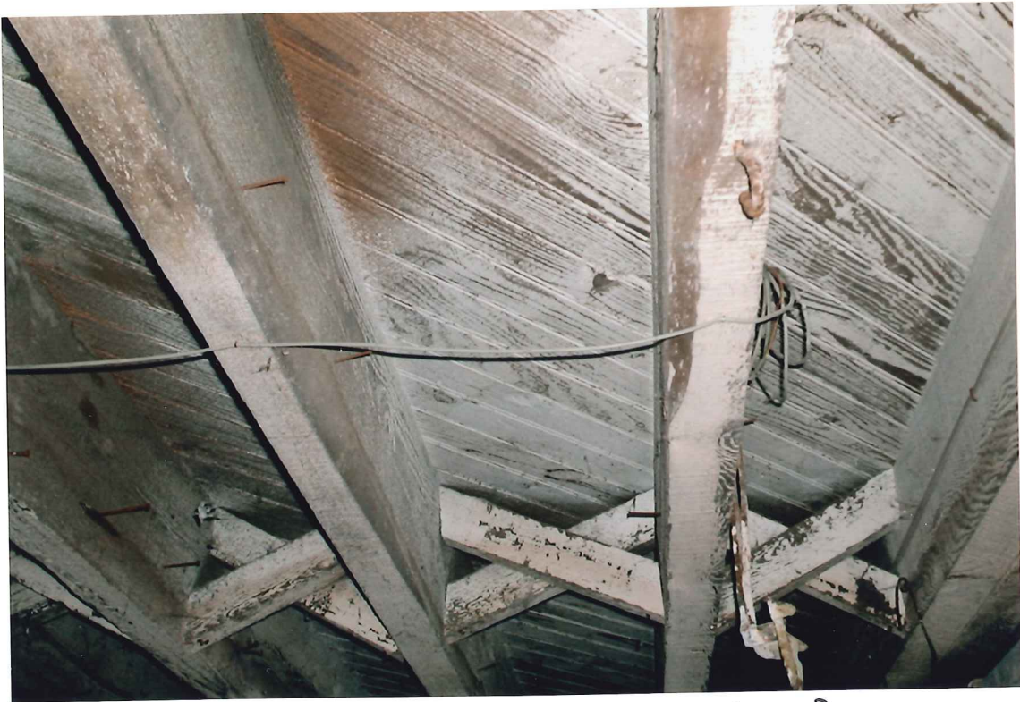
BASEMENT CEILING VIEW - GREAT STURDY CONSTRUCTION
