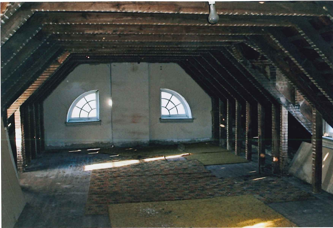
ATTIC - FACING WEST
