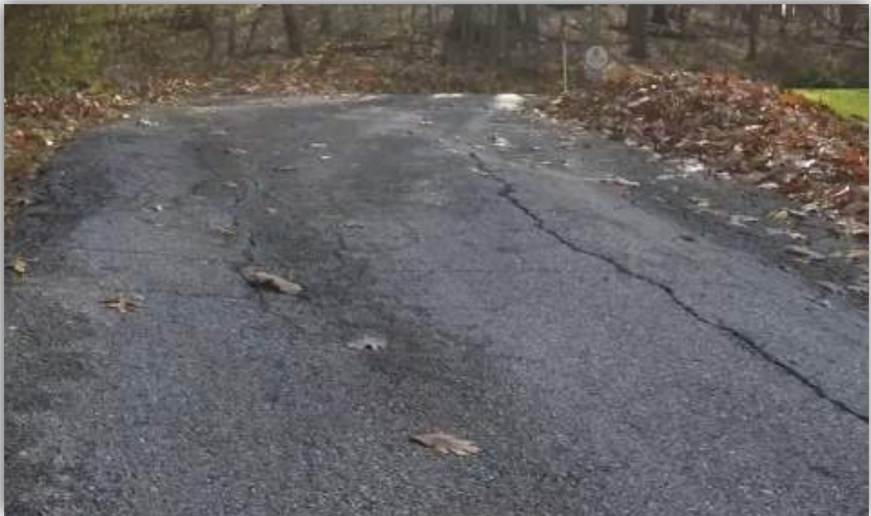
Jewell Avenue – Rutting and Cracking at South End, 7 Score
