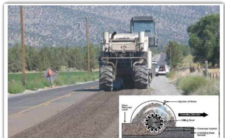
Figure 8: Full Depth Reclamation Construction
