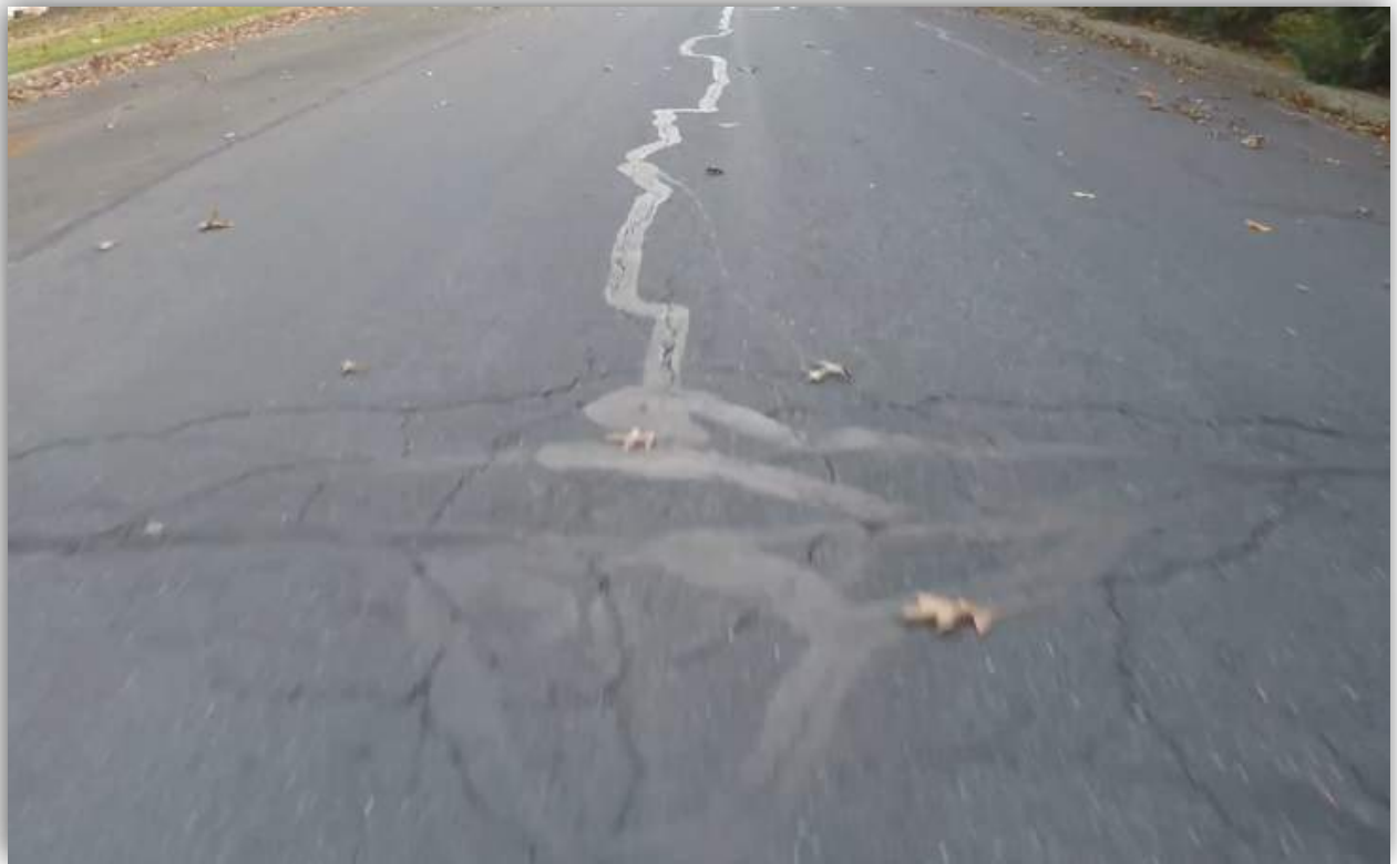
Glen Ridge Drive – L&T Cracking, 7 Score
