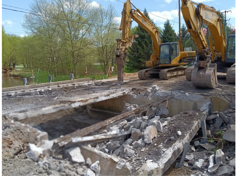
Municipal Drive Bridge Demolition
