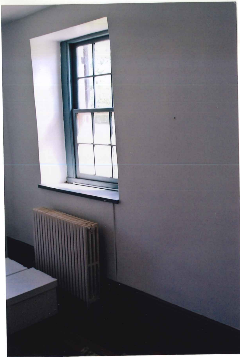
SECOND FLOOR REAR EAST WINDOW
