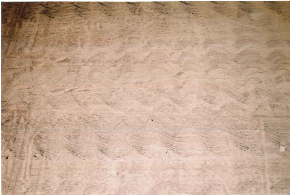
STAIRWAY ART "DECOR" ON CEILING AREAS
