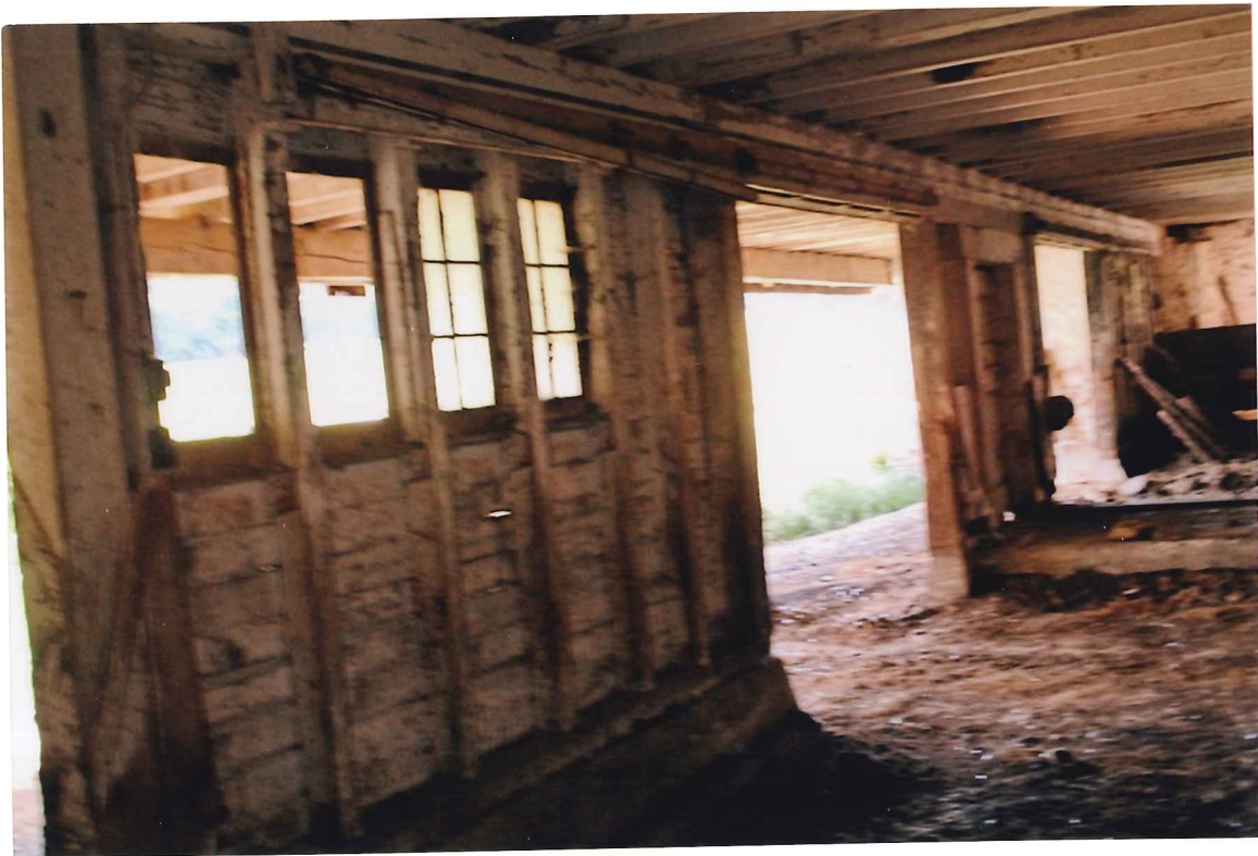
FRONT OF LOWER LEVEL BARN OPENING GOES TO Paddock
