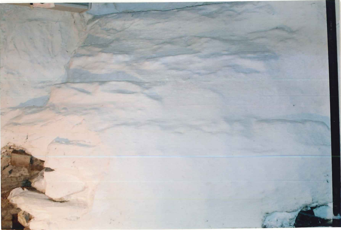
UNKNOWN SUPPORT IN BASEMENT REAR ROOM - EAST SIDE
