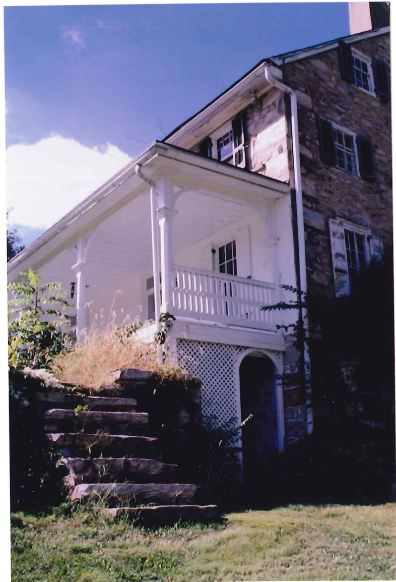
EAST SIDE OF PORCH WITH HUGE STONE STAIRWAY
