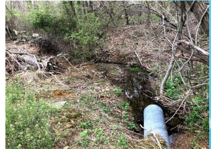
Swale discharging into a tributary to West Branch Brandywine Creek
