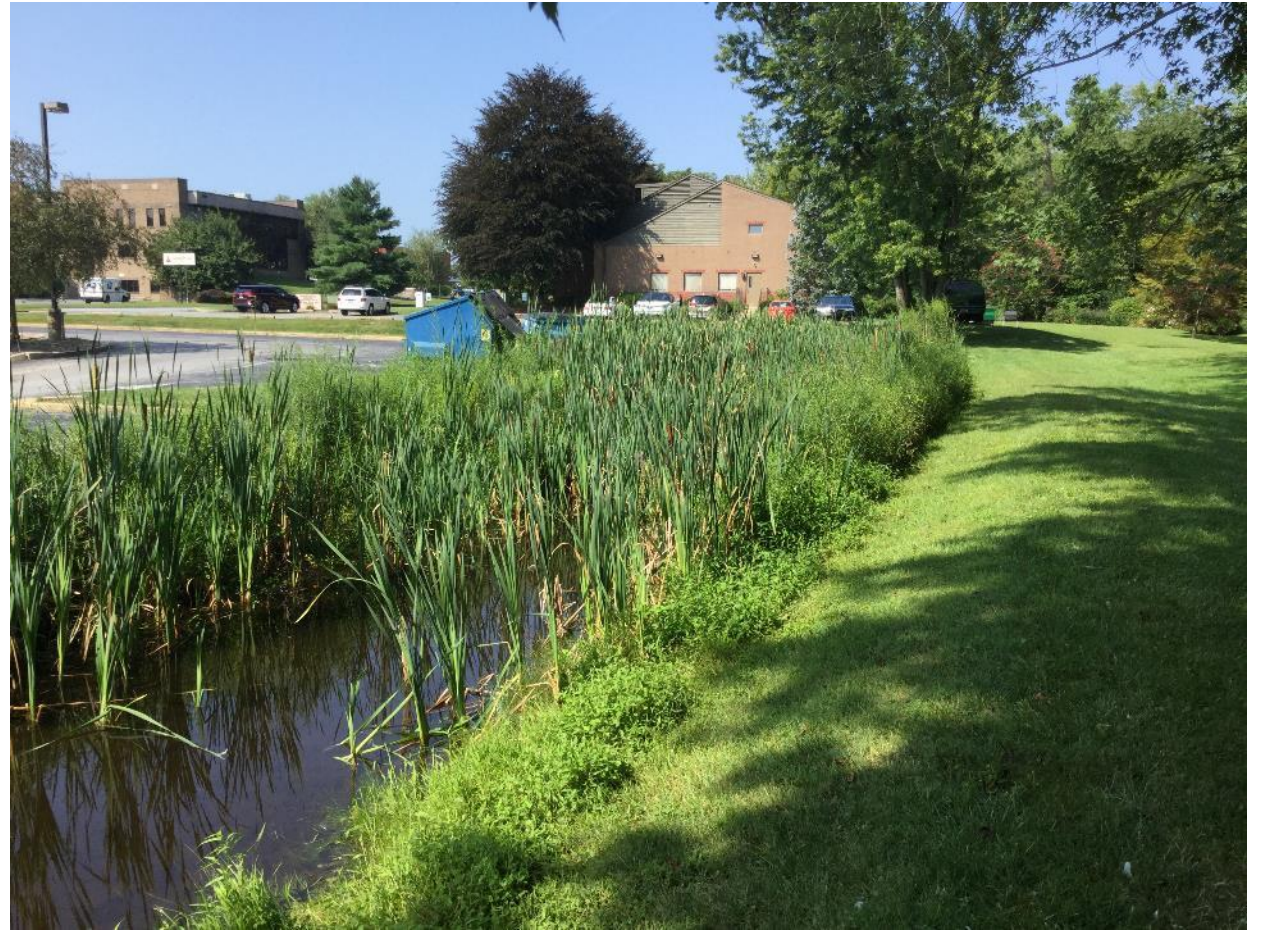
Stormwater Management Facility - N Baily Rd
