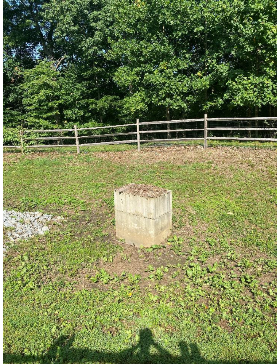
Stormwater Management Facility - Pippen Dr
