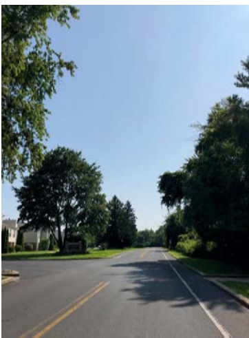
Above: The existing conditions looking east on G.O. Carlson Boulevard toward Park Drive.
