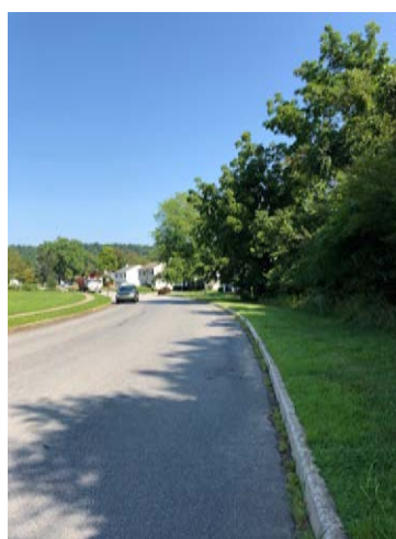
Above: The existing conditions looking north on Park Drive just after the intersection of Park Drive and G.O. Carlson Boulevard.
