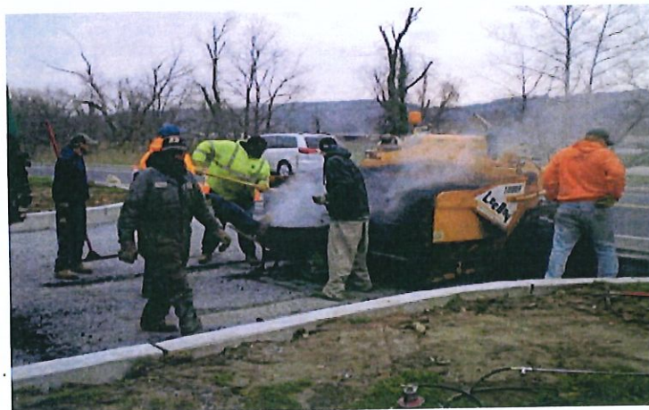
Township Crew Constructs Access Drive at Municipal Complex
