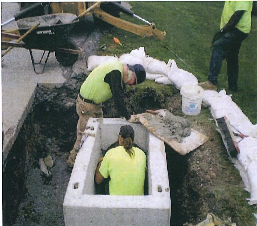
Highway Crew Reconstructing Storm Inlet
