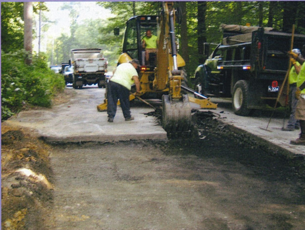
Highway crew reconstructing S. Bailey Rd.
